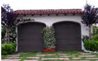
Pairing of Single Car Garage Doors to Appear as One Larger Garage
