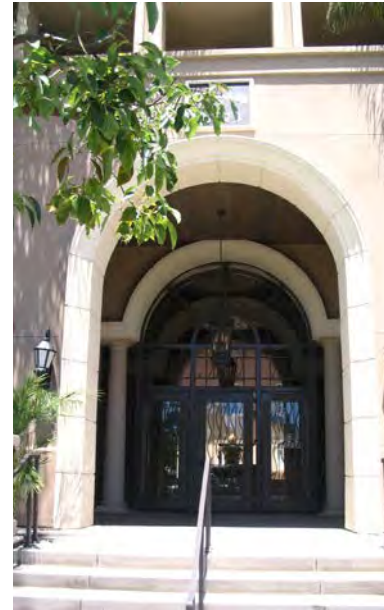
Enhanced Building Entry toward street
