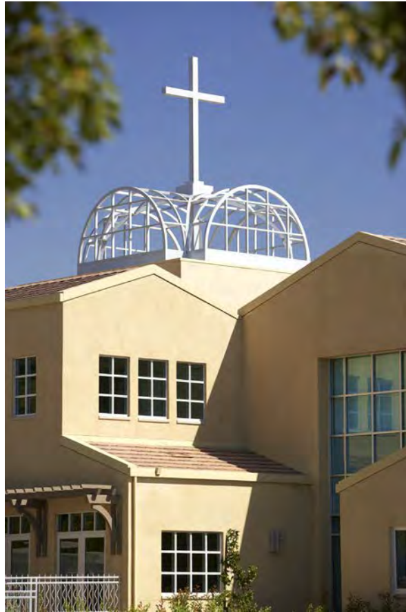
Varied Roof Forms
