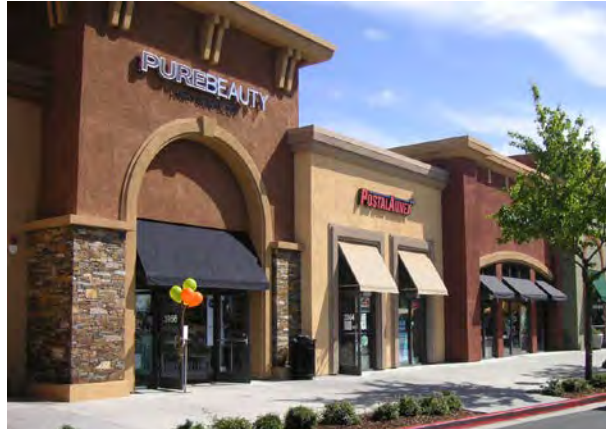
Example of vertical roof breaks, color and material changes, wall plane projections, and architectural elements to create interest and distinguish individual units
